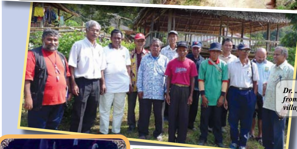
Now: the new bridge suspended from concrete twin towers
